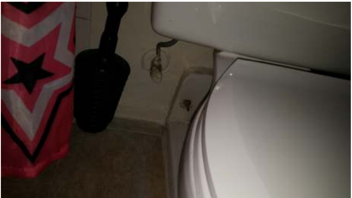
Photo 2: Typical repaired drywall behind the toilet.
