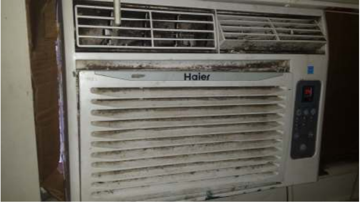
Photo 3: Typical dirty condition of window AHUs
